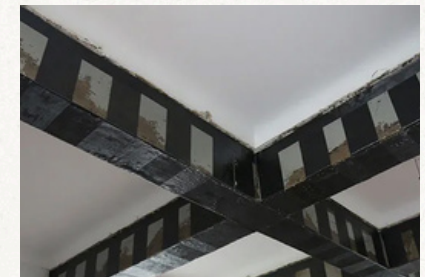
Fiber Reinforced Polymer Jacketing
