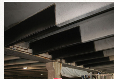
Strengthening Works – Carbon Fiber
