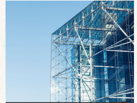
Steel Structure works
