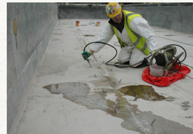
Cracks Injection
