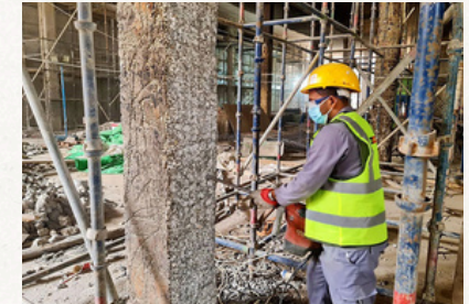
General Concrete Repairs
