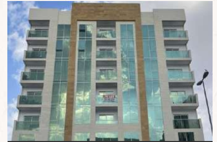
Residential Build. Muwailah
