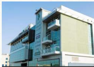
Al Khoory Courtyard
