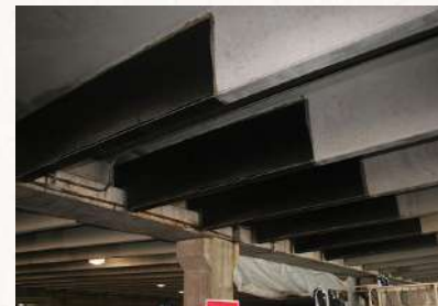
Strengthening Works – Carbon Fiber
