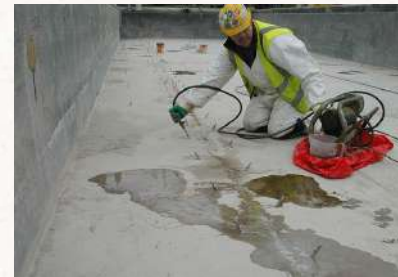
Cracks Injection
