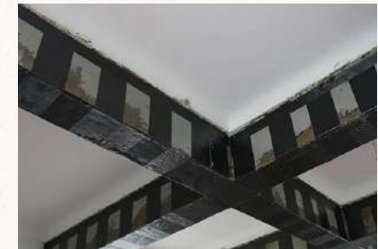
Fiber Reinforced Polymer Jacketing
