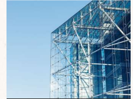
Steel Structure works
