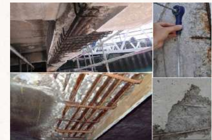
Reinforcement Rust Protection & Repairs
