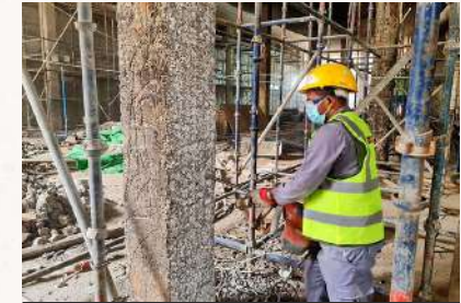
General Concrete Repairs
