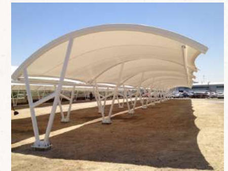
Car Park Sheds
